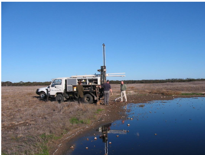
Figure 4. Drilling on edge of soak at site RO3
